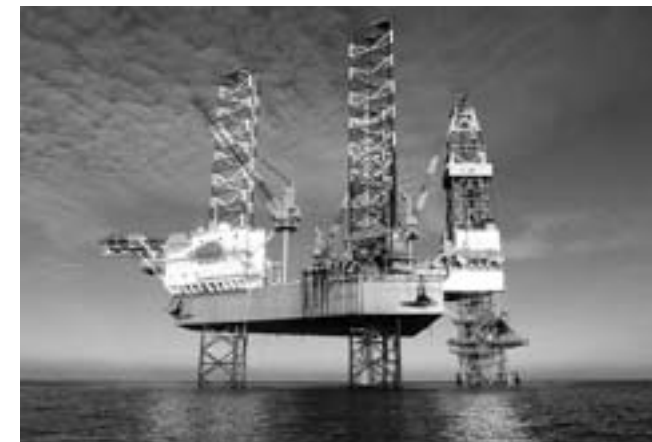
Jack-up rig is a typical construction that requires high performance filler metals with high impact toughness and low crack susceptibility. (Photo courtesy of Kansai Design Co., Ltd., Japan)
