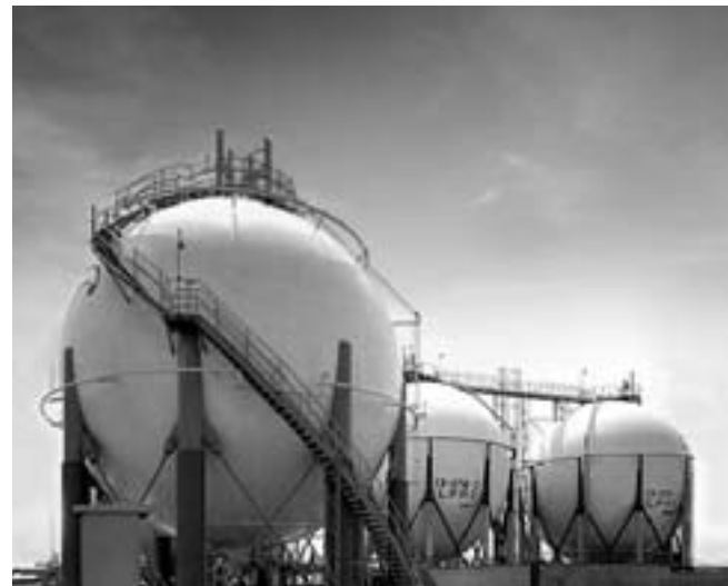
Some types of LPG storage tanks use ASTM A537 Cl.2 steel having a minimum tensile strength of 550 MPa, and LB-62L is one of the most suitable covered electrodes for this steel.
