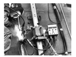
Figure 11: The SEGARC process being used for EGW of a vertical hull joint.
