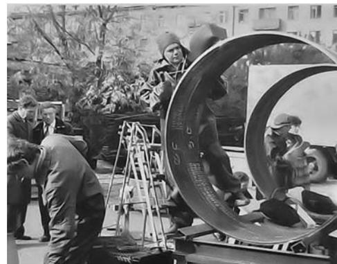
Figure 12: Welding test of covered electrodes on pipeline segments in the then Soviet Union in 1982.
