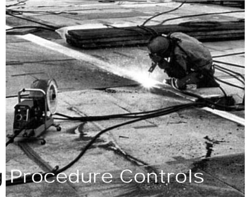
The cargo tanks and piping systems of chemical tankers use special grades of austenitic and duplex stainless steel to resist their corrosive cargos. Such particular stainless steels require special consideration and handling to obtain successful welding results. Following Part 1, “How to Select Stainless Filler Metals,” Part 2 of this two part series on welding chemical tankers discusses the essential factors in welding procedure controls.
