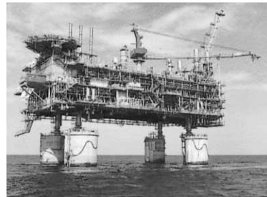
Left: The production platform for the Malampaya Deep Water Gas-to-Power project, for separation and condensation of the gas from water (Courtesy of Shell Philippines Exploration B.V. and SMOE)
