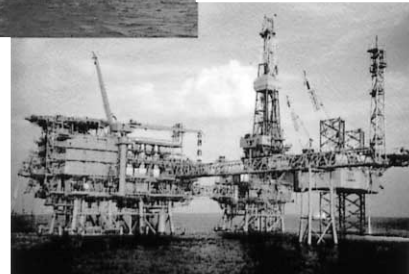
Right: The Balal-PJ Platform consists of process and living quarters platform and wellhead platform
